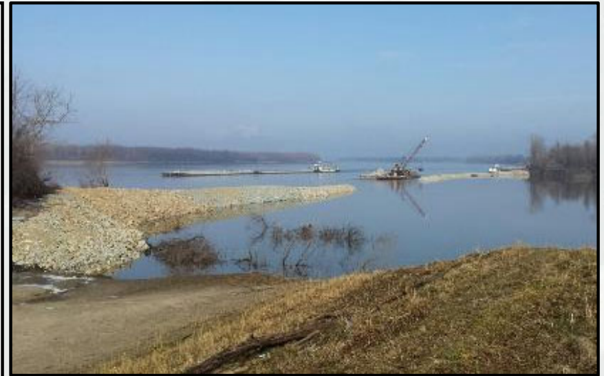
Construction Execution - Bankline Restoration at Dogtooth Bend (Len Small)
